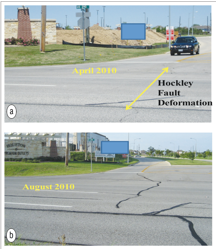
Figure 13. Recent pictures of Hockley fault at Highway 290 Frontage and Fairfield Falls Way roads: (a) taken in April 2010 and (b) taken in August 2010. Note the development of the tiny cracks in (a) into significant ones in (b).
