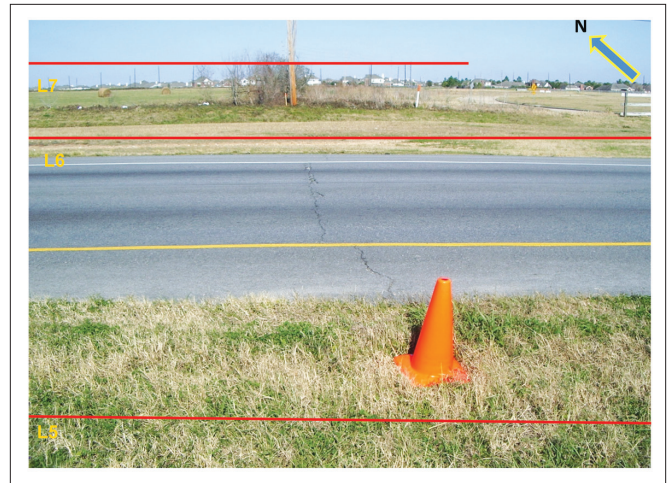
Figure 4. A picture showing a significant crack on the westbound lane of Highway 290 prior to the construction of a shopping mall. The picture was taken facing north. Approximate locations of resistivity profiles L5, L6, and L7 are shown.
